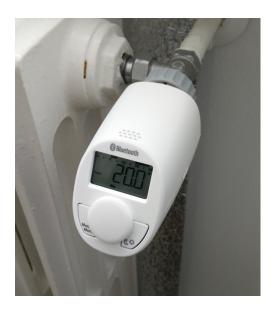
Fig. 1: EQ3 Eqiva valve on a radiator
